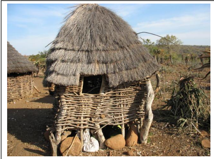
Figure 7: A different traditional design of the maize crib from Lubulini in the Lowveld of Swaziland. The maize crib is short and thatched. The crib is built with local material only.
